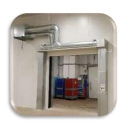
This unique high-pressure air curtain system was specially developed for use for doors between large freezers in combi with big conditioned front rooms. Here, the function of temperature and humidity separation is split into two individual functions. The temperature separation is ensured with a predefined outblow angle of the separation air jet against the natural flow direction.
