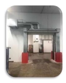
As standard, this basic system is installed on the freezer side. In opposite to the typical Masterveil approach, the tailormade length is reached by combining standard modules.
